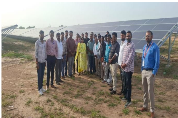
Visit to Solar Power Plant
